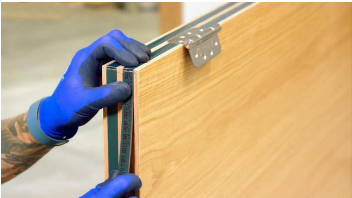
Figure 5: Generic example of fitting intumescent strip
