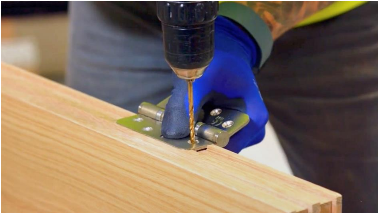
Figure 4: Generic example of fitting the hinges
