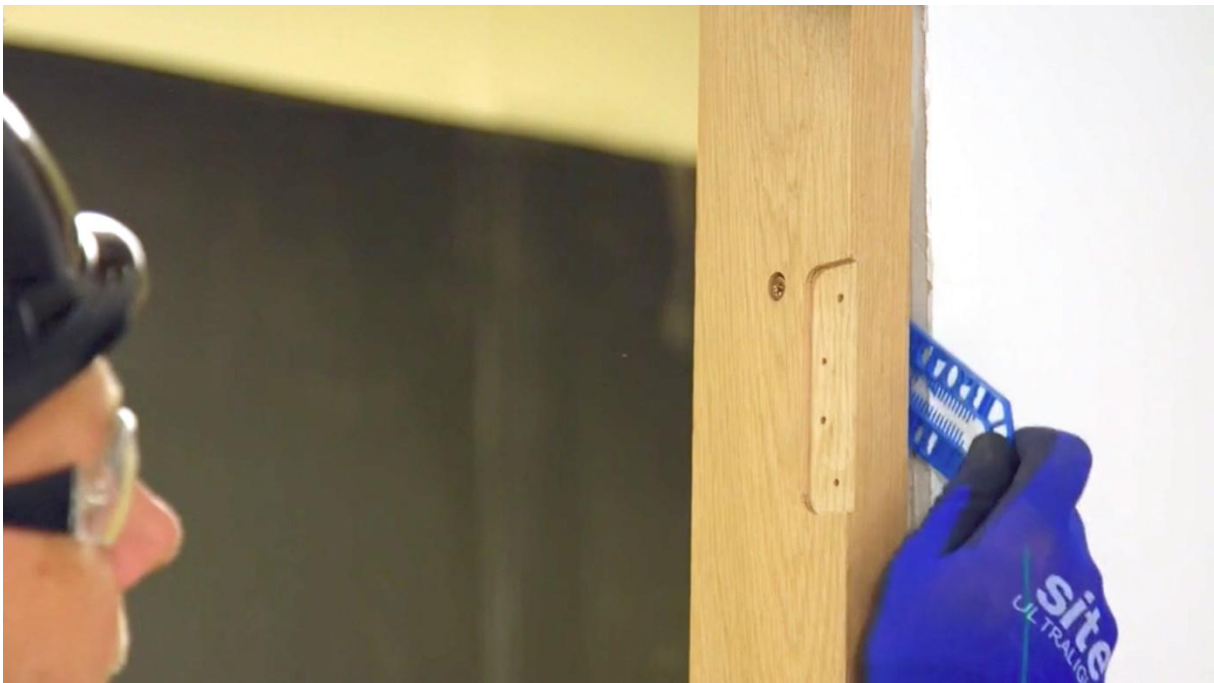
Figure 5: Generic example of install packer
