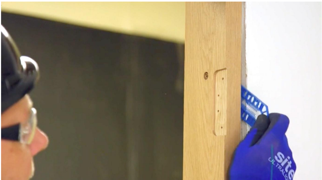
Figure 5: Generic example to Install packer
