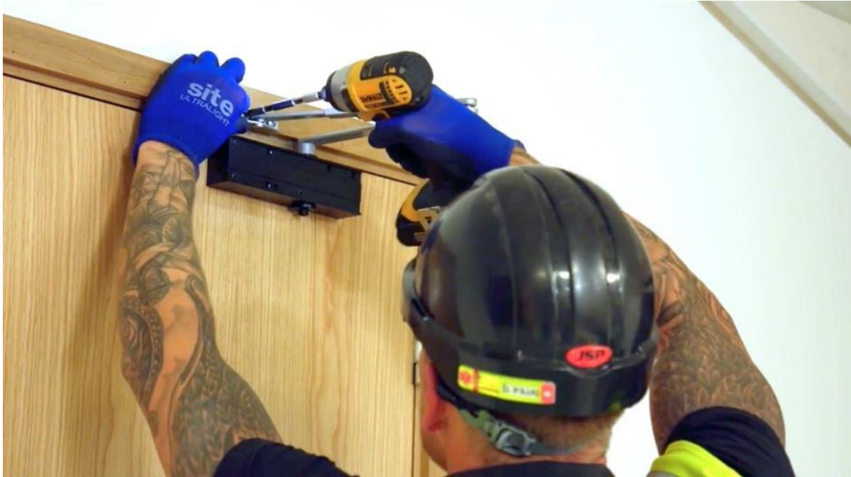
Figure 6: Generic example of installing ironmongery
