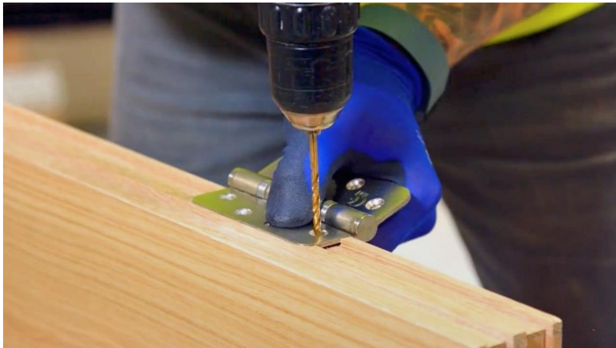
Figure 4: Generic example of fitting the hinges
