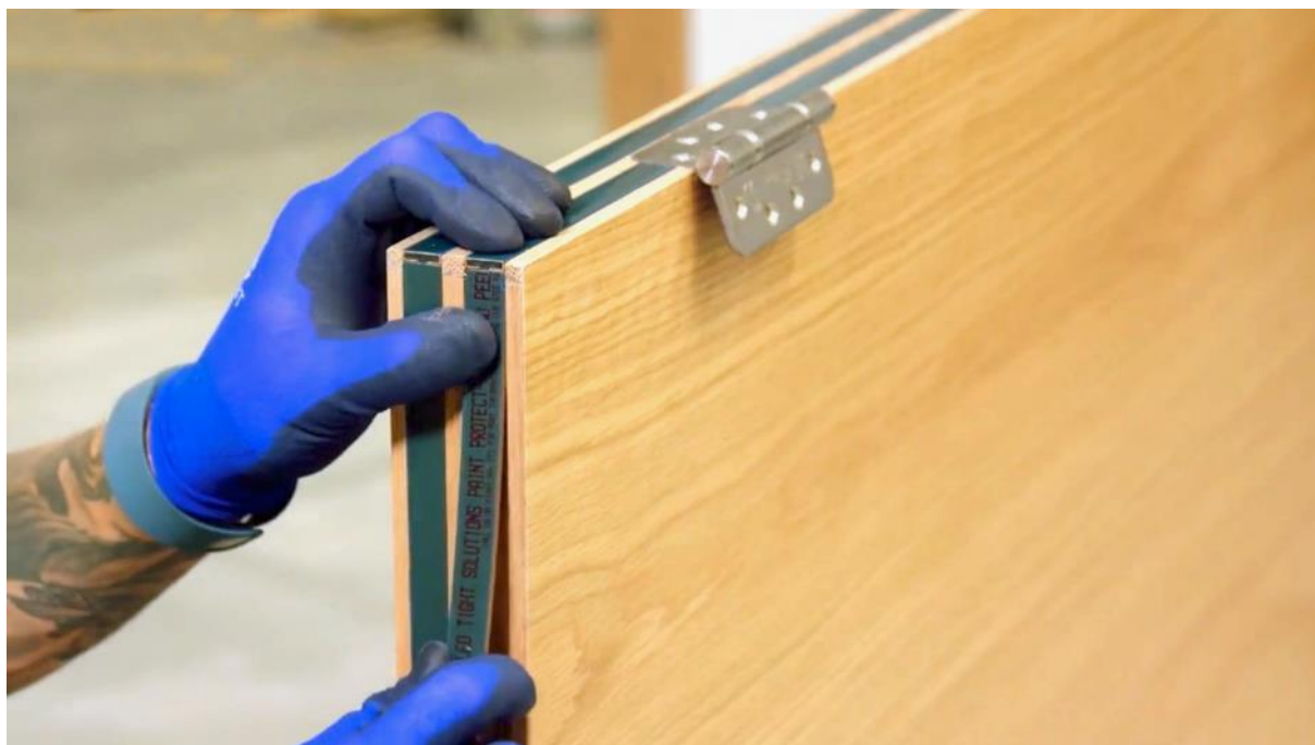
Figure 5: Generic example of fitting intumescent strip
